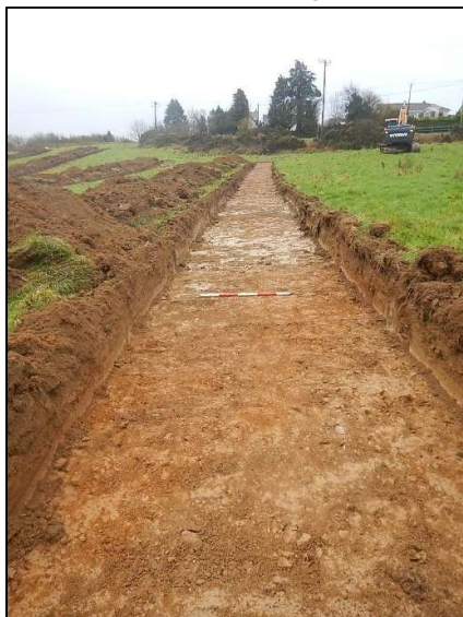
Trench 14, looking S
